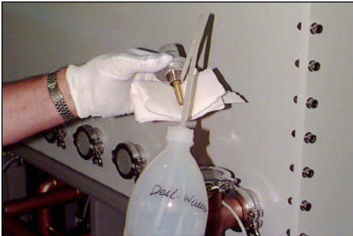
Cleaning the sensor with distilled water
